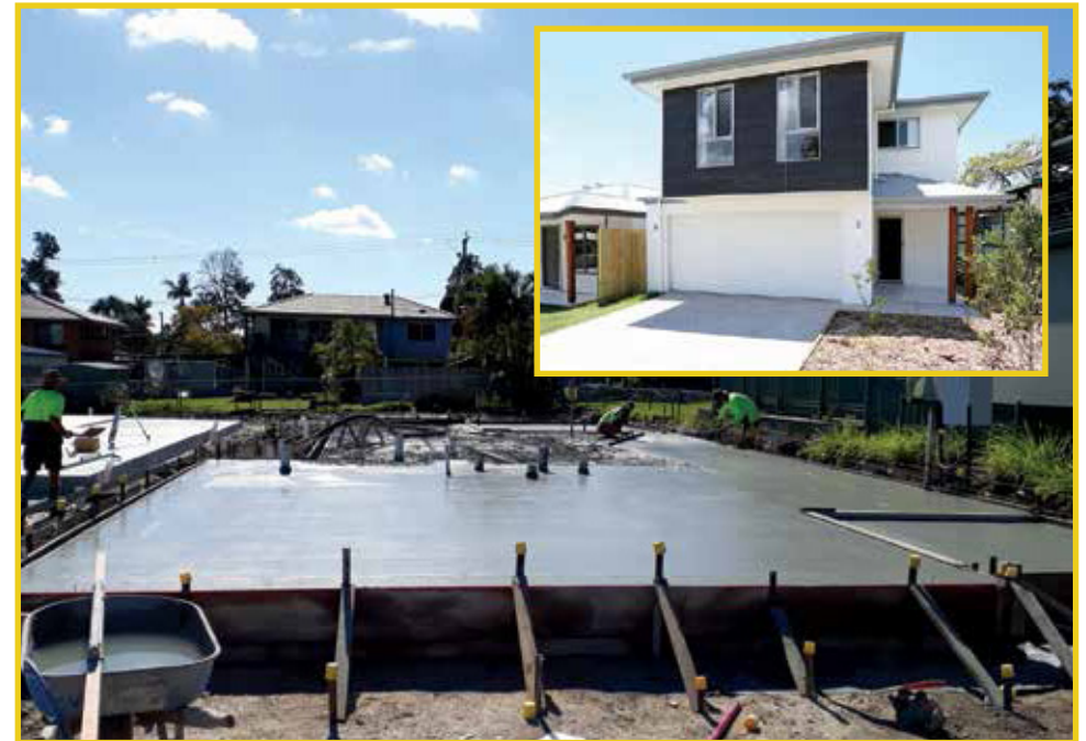
(Pics: main - initial slab poured: inset - completed house)
